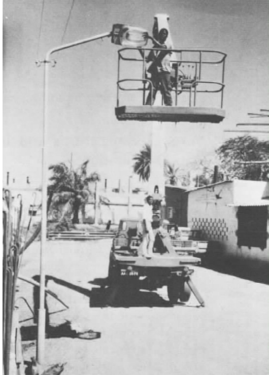
A utility crew in Luanda fixes a street lamp.
